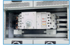
NZM2 circuit breaker with removable neutral link.
