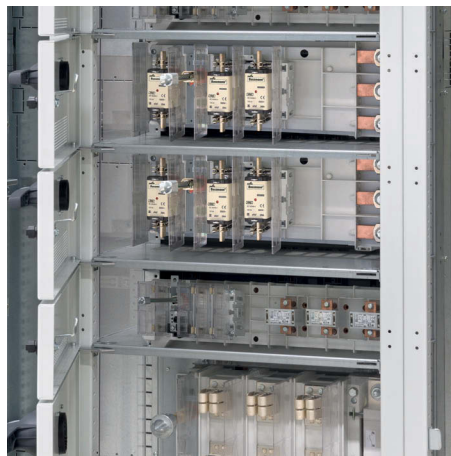
Form 4a with type QSA fused combination switches.
